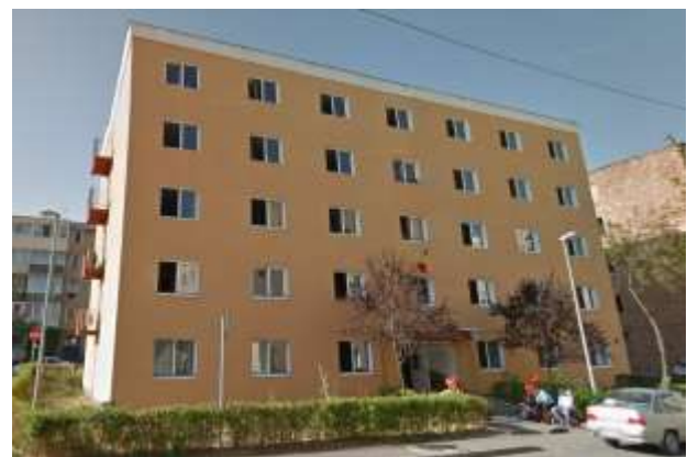
Figure 1: Photo of the precast-concrete walls case study in Brasov
