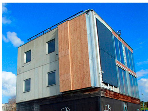
Figure 14. BERTIM system installed in a section of the west façade at the KUBIK by Tecnalia test facility.
