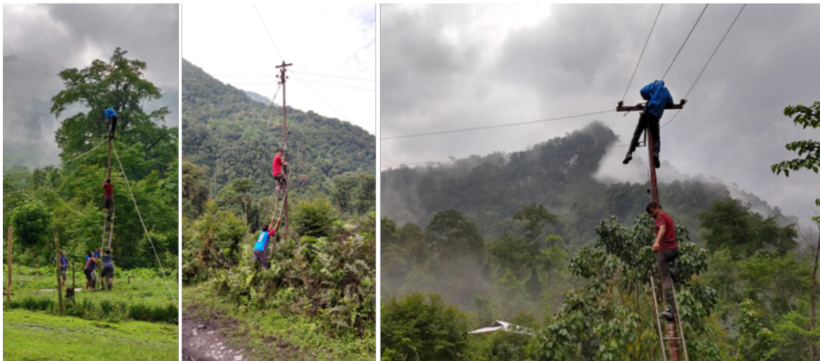
Figure 13.14: Installation of overhead cables.[93].
