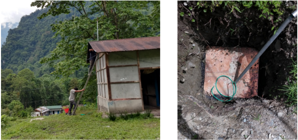
Figure 13.15: Installation of the lightning arrester and the copper plate.[93].
