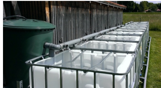
Picture of the IBCs setup with the collecting tank including the filter unit
