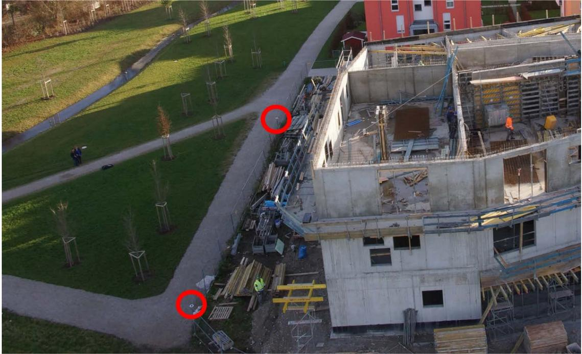
**Figure 16** Registration of SfM-based point clouds using geodetic markers.
