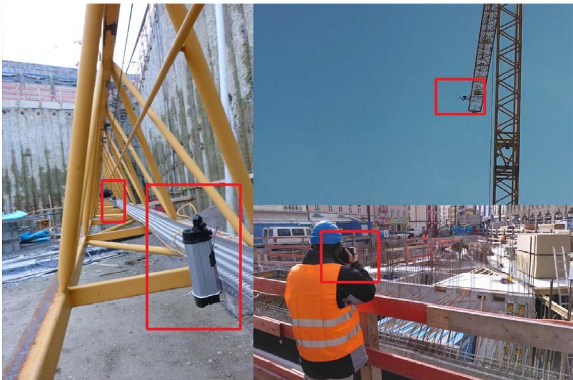
**Figure 15** Proposed methods for image acquisition that were investigated during this research. Left: crane cameras, top right: UAVs, bottom right: manual acquisition.
