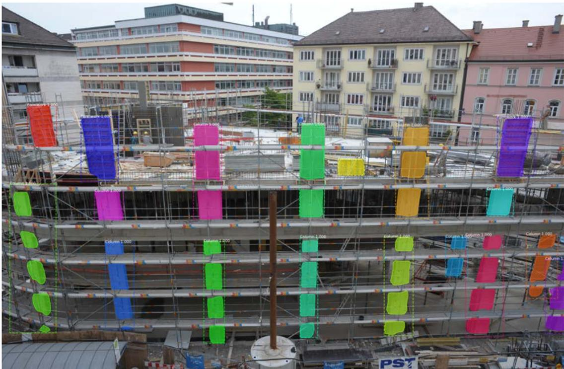
**Figure 64** Detected construction elements on an image taken during monitoring.
