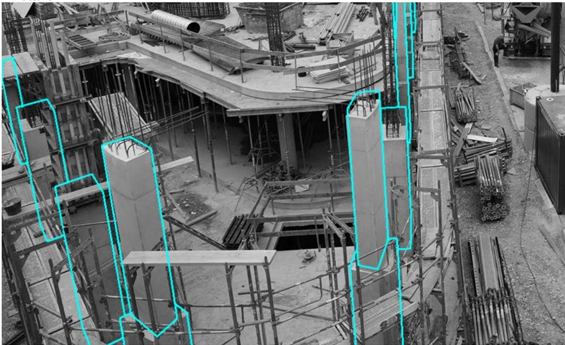
**Figure 60** Sample sub-set of auto-labeled columns in one picture from a construction site.
