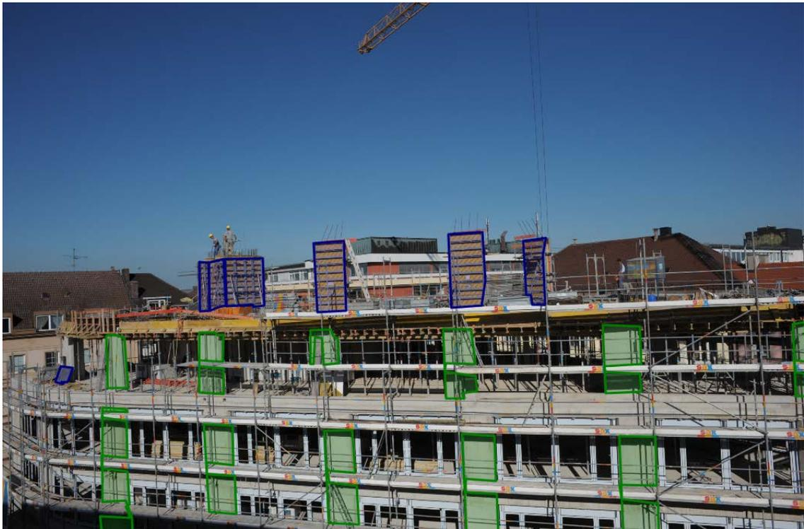
**Figure 42** Sample image of the labeling process. Displayed are the labeled formwork (blue) and column (green) elements. During this research, Labelbox (Labelbox, 2020) is used for labeling.
