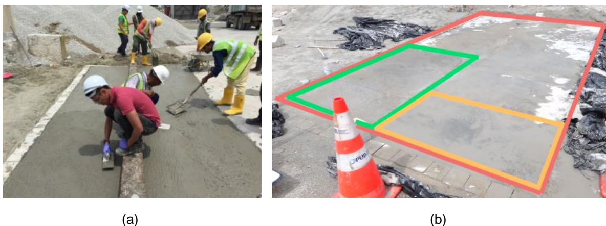
Figure 8.2 Finishing stage (a) surface levelling, (b) results with cast in situ
