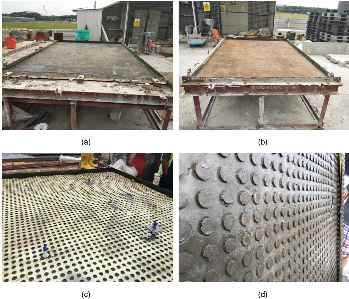
Figure 8.8 Precast method (a) steel mold used for large slab, (b) steel mold used for small slab, (c) silicone mattress with circular holes and (d) circular convex nodes on the bottom surface of slab.
