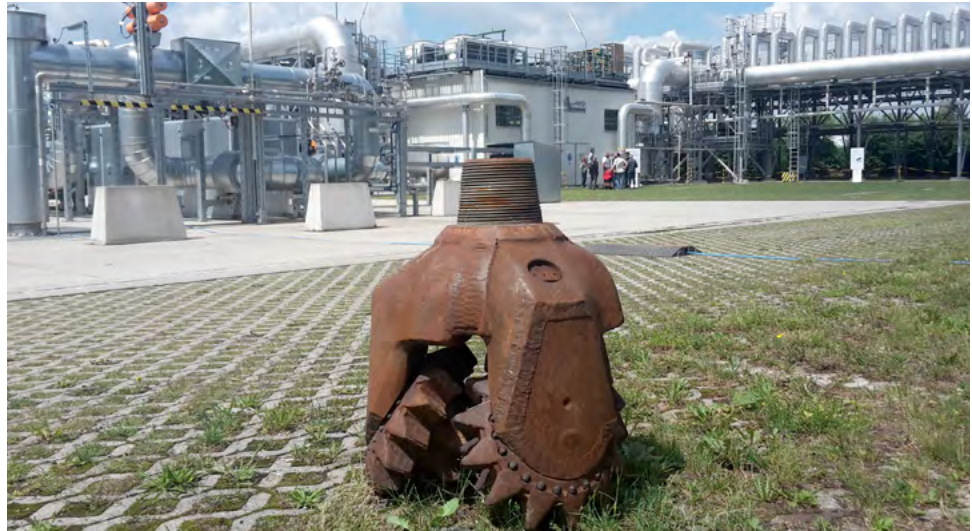
■ Visit of the geothermal plant Kirchstockach. In the foreground a drill bit can be seen, in the background the geothermal power plant. Source: Geothermal Alliance Bavaria, TUM.
