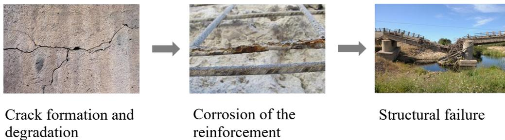
Figure 1. Degradation process of concrete supporting structures.
