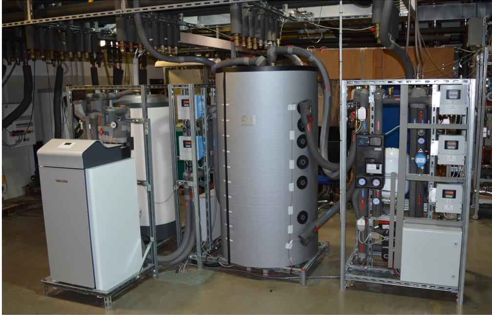
**Figure 2.2:** The three modules and the heat pump installation in the lab.
