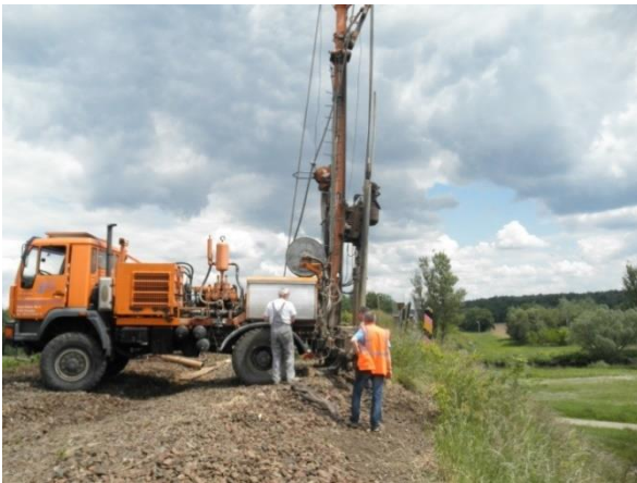
Figure 4.1: Drilling rig on the traffic embankment (named Neißedamm ), Eastern Germany
