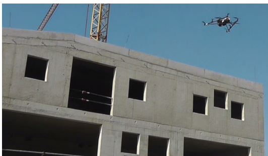
Figure 1. Octocopter with Nex-7 camera mounted in front of the construction site
