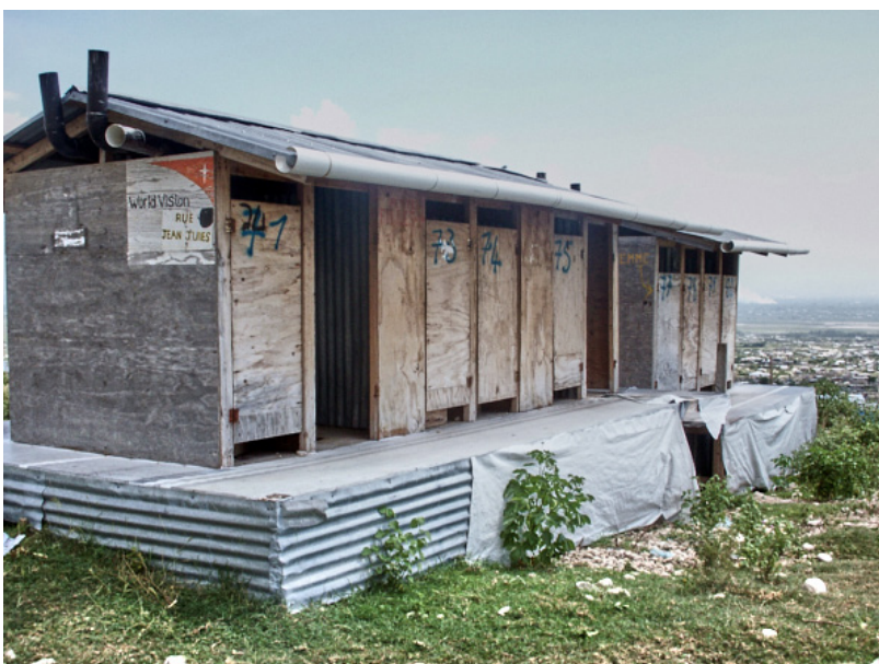
Fig.29: Filled with feces, many community latrines are unusable, 2012 (Courtesy of Gökçe İyicil/Fidan)
