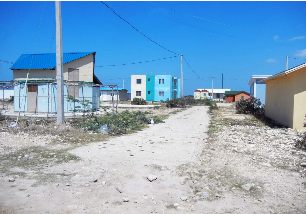
Fig. 34: Degraded building exposition, Zoranje 2013
