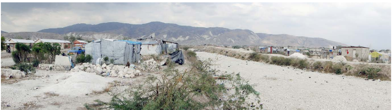
Fig. 16: Camp Corail, Sector 4 (left); new settlers construct in regular flood zone on the river banks of Ravine Madaniel
