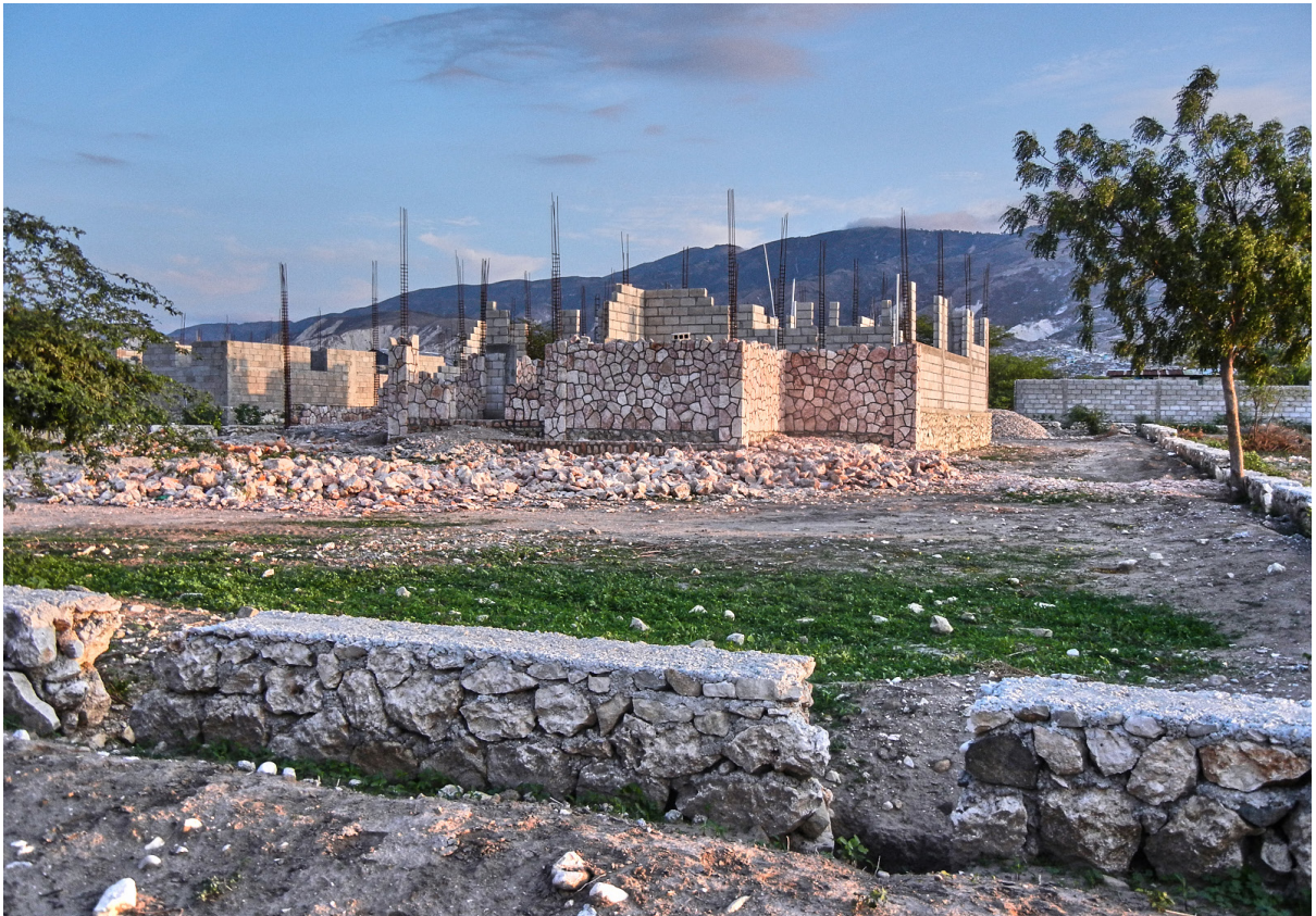
Fig. 41: Construction of a magnificent building, Bas-Onaville
