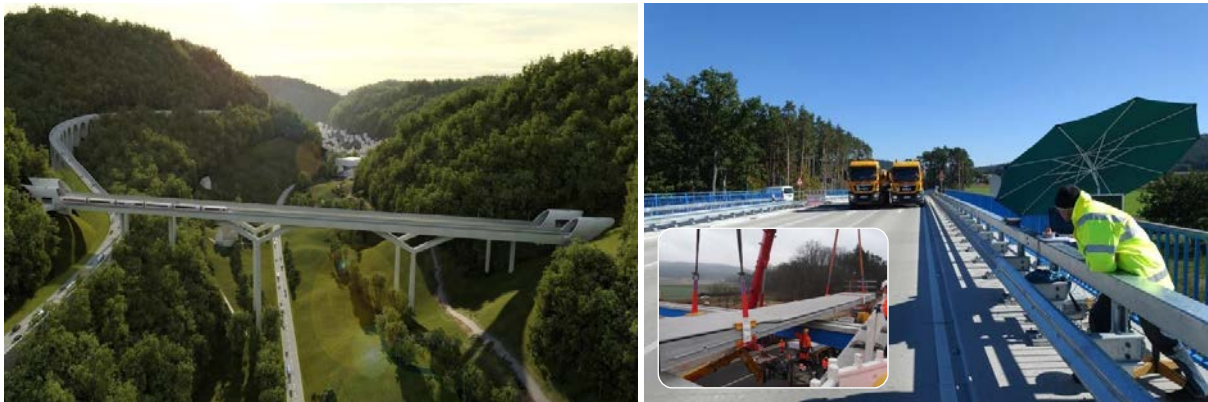
Fig. 2. (a) Filstal viaduct (computer animation, DB Netz AG); (b) Greißelbach bridge with segmental roadway slab (here: loading test)
