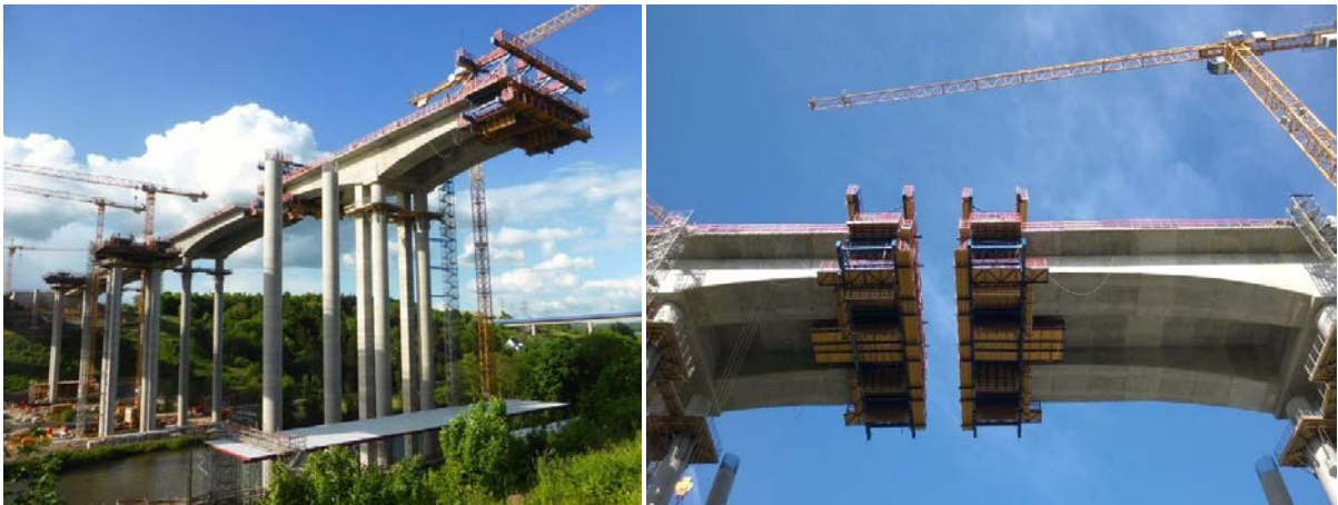
Fig. 1. Lahntal bridge, (a) balanced cantilever erection with auxiliary pier; (b) twin-box cross-section (width 21.44 m) before closure at midspan
