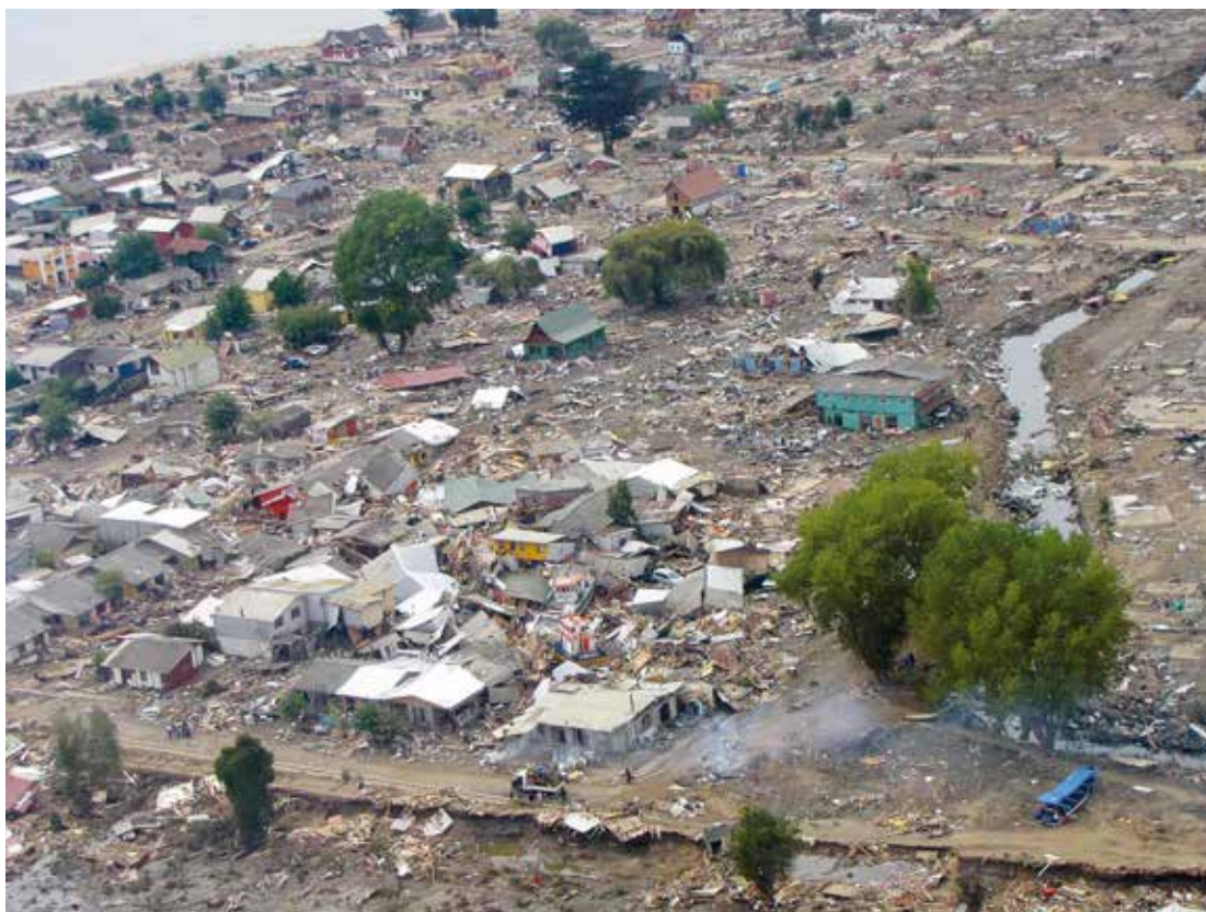
Figure: 1 Aerial Assessment of Concepción (02 March 2010) after an 8.8 earthquake followed by tsunami on 28 February 2010. © International Federation of Red Cross in Flickr
