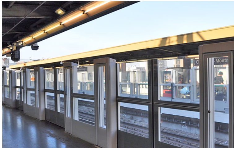
Figure 9.1: Platform screen doors installed in Paris
