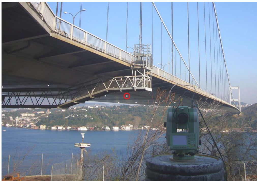
Figure 4.6 – Fatih Sultan Mehmet Bridge seen from observation pillar with highlighted LED targets. The red circle indicates the IATS observed target
