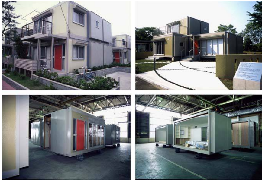
Figure 2. Sekisui Heim's legendary M1 was the first prefabricated housing model which reached a annual production of over 3,000 buildings/year over several years
