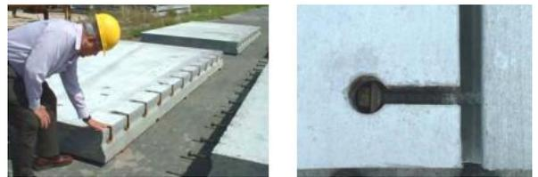
Figure 4-7: Kwik Slab joint interlocking system (Buch, et al., 2012)
