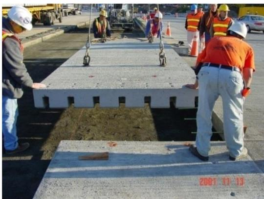
Figure 4-5: Dowel bar slot at the bottom of the slab (Buch, et al., 2012)
