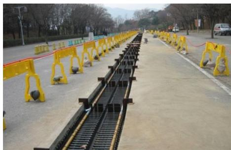
Figure 3-16: The pavement for the W-type power supply rail (3G) ([www.heise.de](http://www.heise.de))
