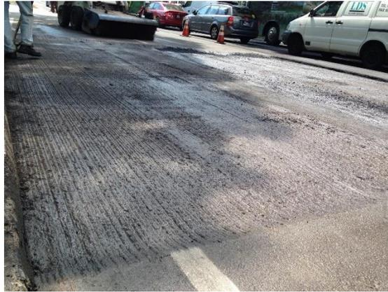
Figure 9-6: Asphalt surface after milling (at Clementi Road, Singapore)
