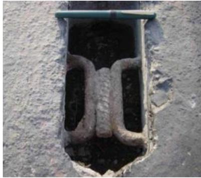
Figure 4-2: Welded lift loop connection (Tayabji, 2011)
