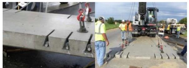
Figure 4-9: Narrow mouth surface dowel slot (Buch, et al., 2012)
