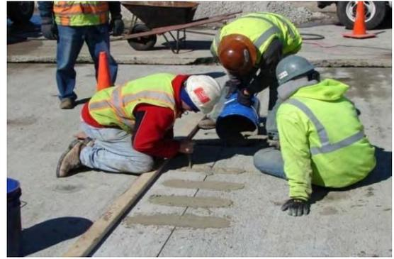
Figure 4-6: Installing dowel bars using DBR method (Buch, et al., 2012)
