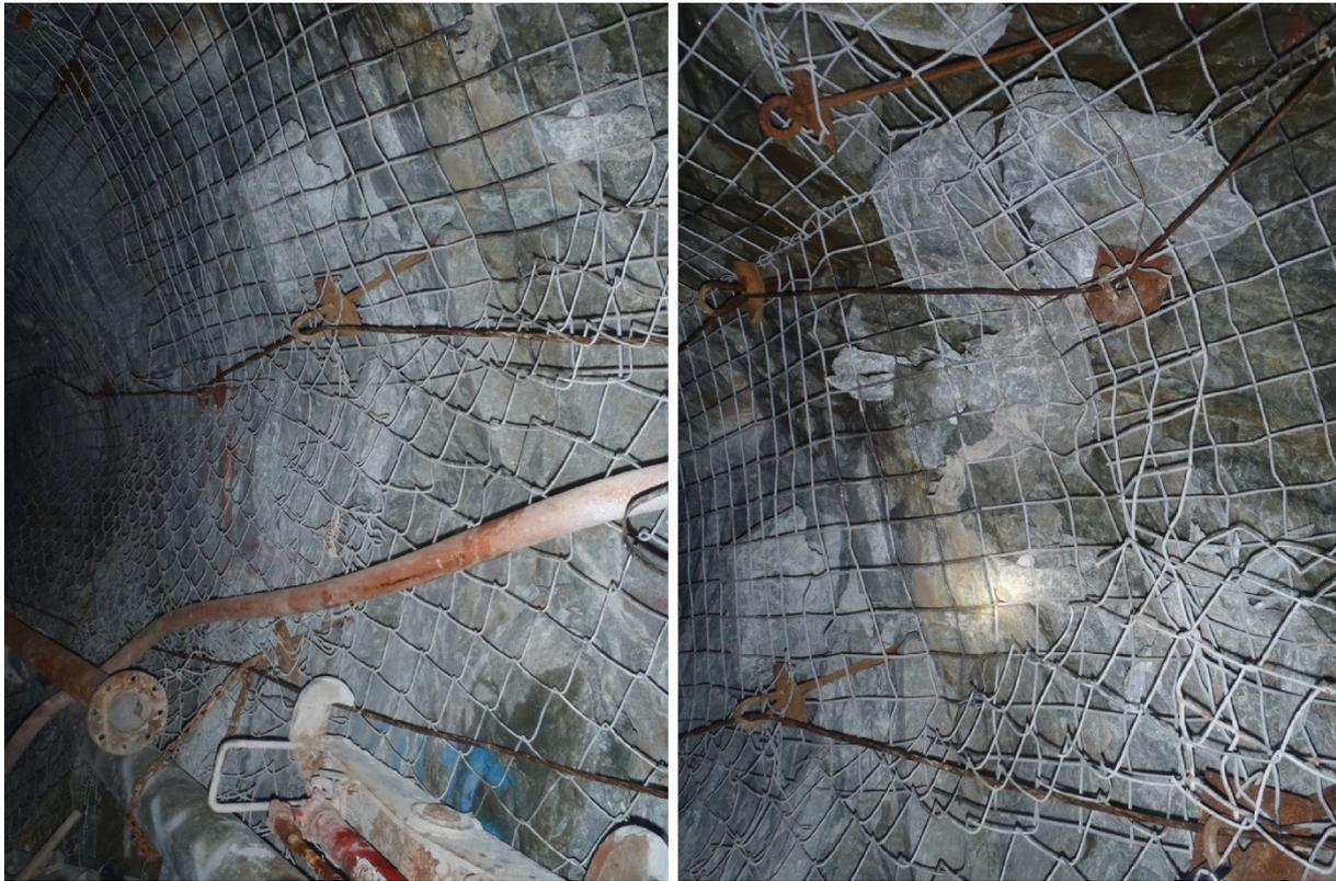
Fig. 130: Stress induced loosening of rock mass at the side walls of the transportation gallery.
