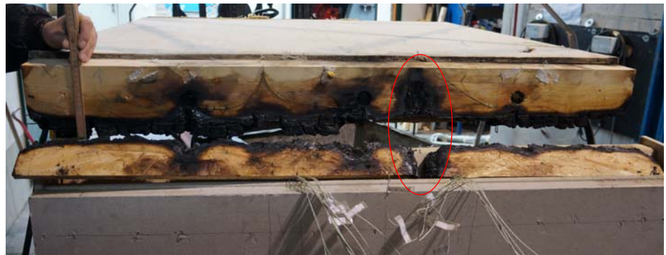
Figure 30 Small-scale fire test – wall-floor – 90 min – almost burn-through between OSB and coupling beam (red circle)
