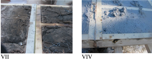
Figure 14: view of jointing area after deconstruction
