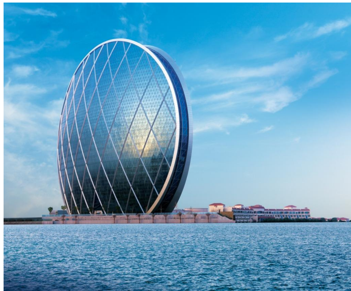
Abb. 3.3: Aldar Headquarters, VAE
