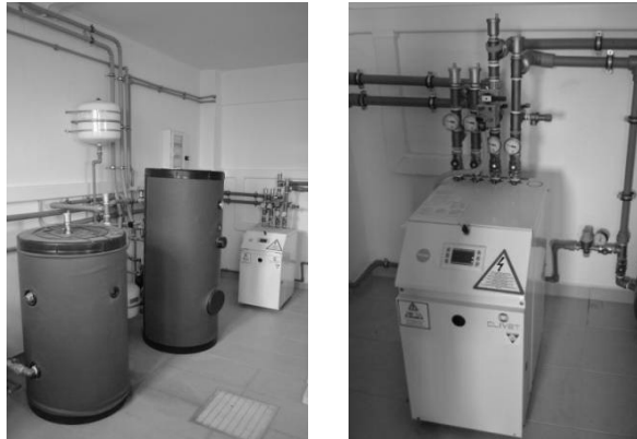
Figure 9: Photographs of the mechanical equipment. a: Buffer tank of 150lt and boiler of 200lt b: The Clivet 51 heat pump (15,7 kW heating capacity)
