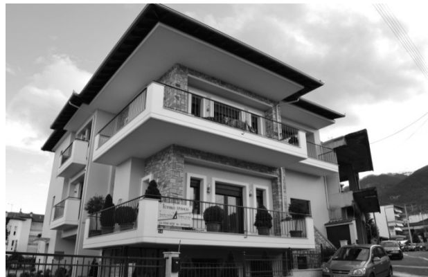
Figure 3: North (and partly east) facade.
