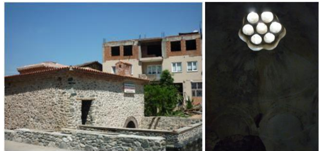
Figure 1: The Demirci Hammam- Bursa, internal view showing the toplit dome of the northern hot room (right)
