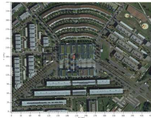
Figure 7: Aerial view of Solar City, Linz, Austria.
