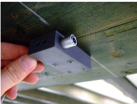
Figure 10: Measuring point on main beam
