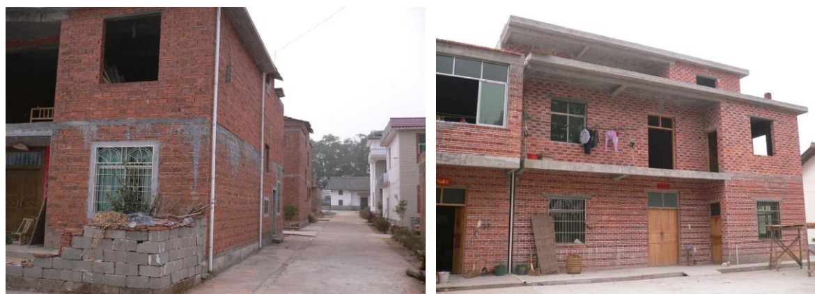
Photo 3: Unfinished New House in Ganzhou
