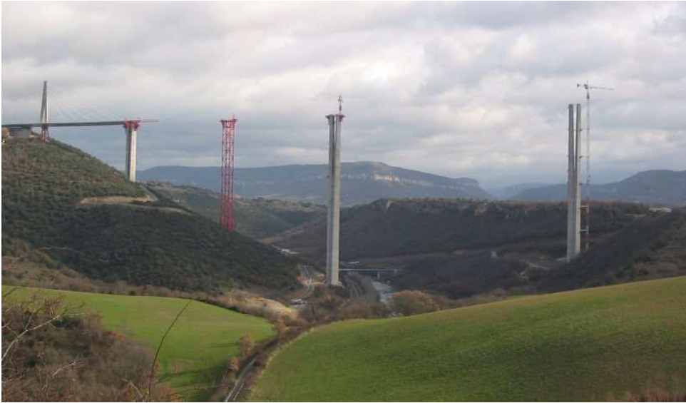
Figure 9.3: Millau Bridge in construction [141]
