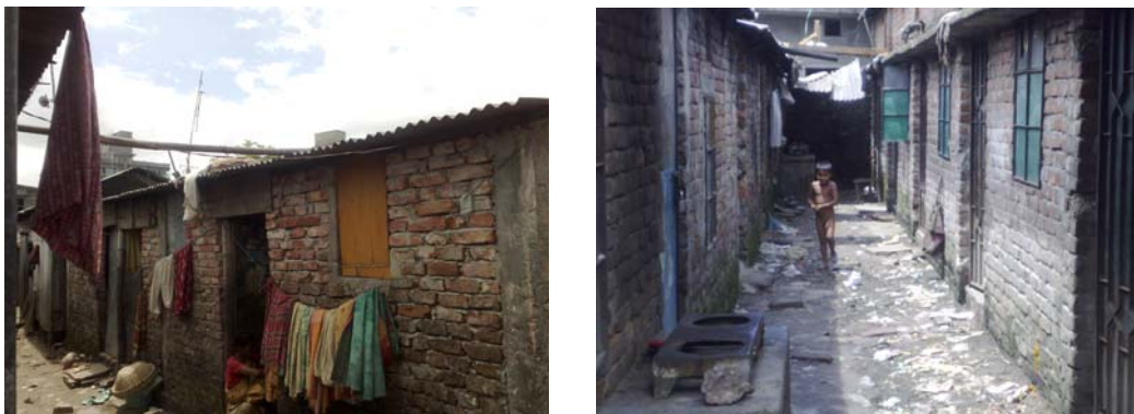
Photo 12 & 13: Building development without planning regulations
