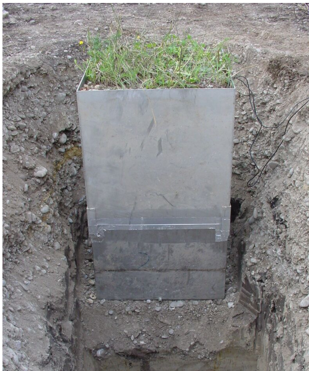
Figure 6 Installation of Lysimeter 3 at the field site.
