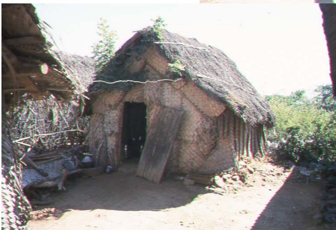
Fig. 3.10: Typical houses in the study area: out of bricks and tiles (above), with walls out of clay and a grass roof (middle) and made from coconut tiles and grass
