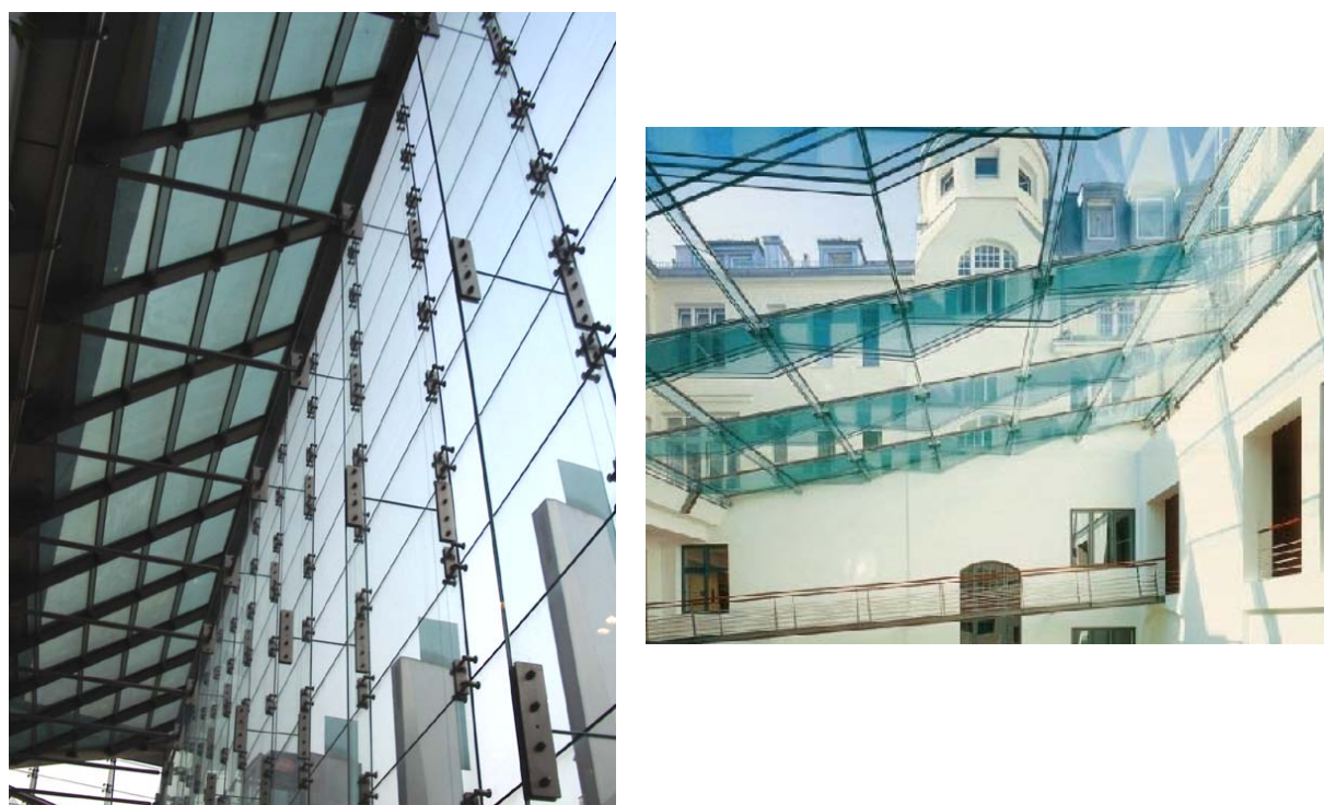
Figure 1.1 Examples of loadbearing glass structures
