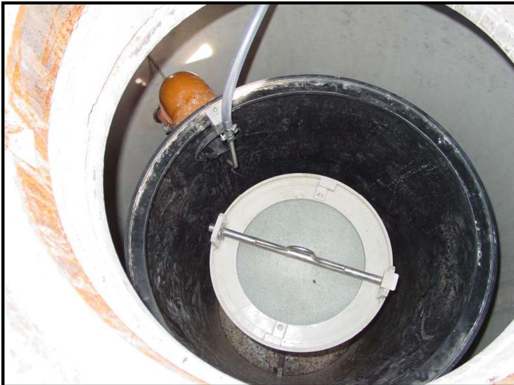
**Figure 23:** Filtration tank with the zeolite cartridge.
