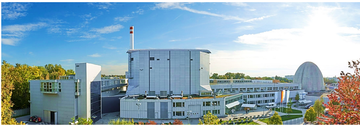
Figure 1.2: The FRM II (middle) with the dome of its predecessor FRM on the right.
