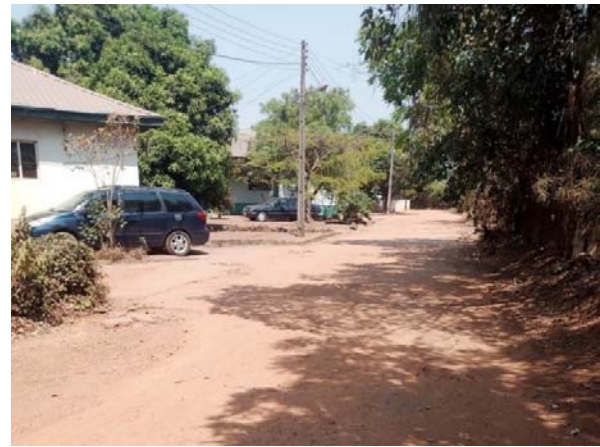
Fig. 3 A street in a government housing property in Enugu with unpaved access road and no drainage channels
