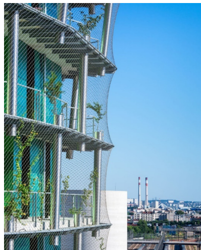
Figure 4. Tube-like planters with small trees on the Tour de la biodiversité after completion (Pierre L'Excellent 2016).
