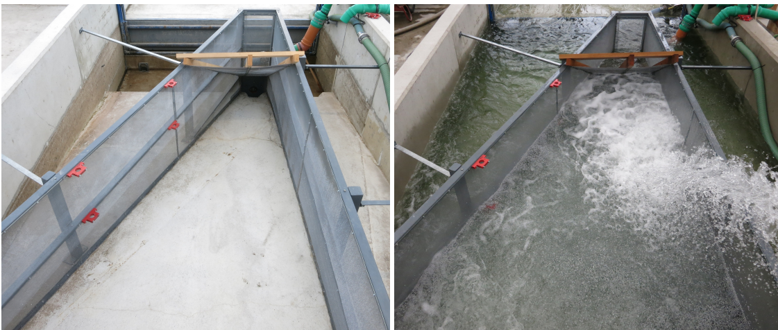
Figure 20: Sediment trap, dry (left) and during operation (right)
