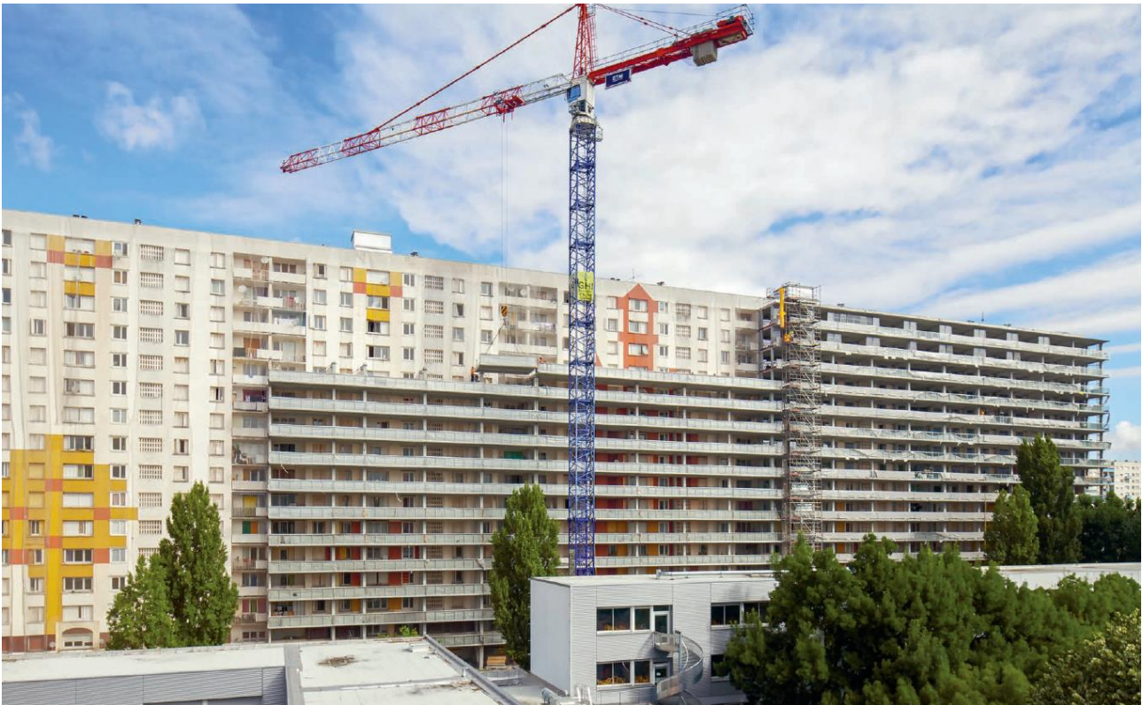
Figure 44 – Photo during the assembly phase of the renovation with extensions of the 530 dwellings in Bordeaux [94]
