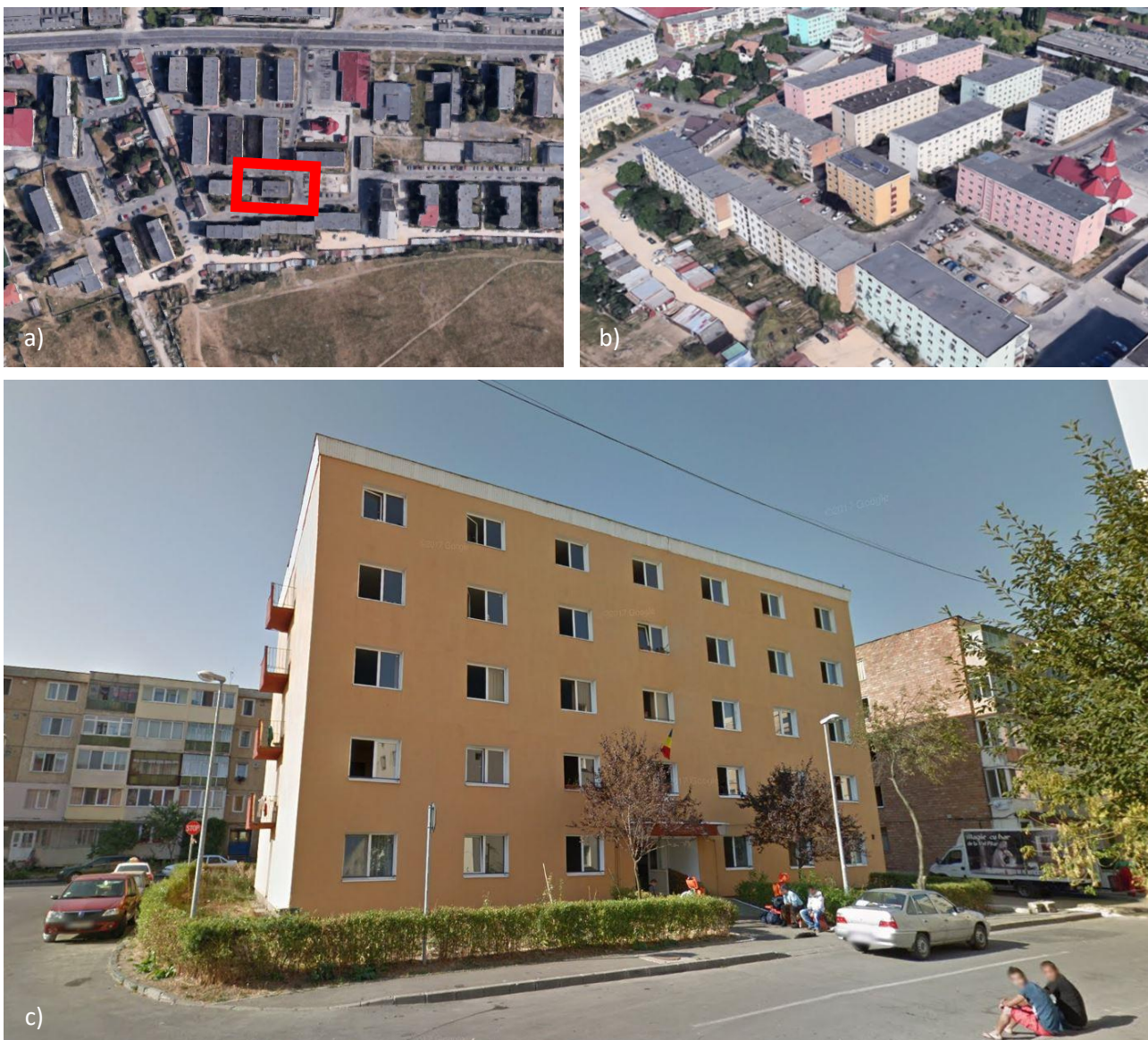
Figure 160 – a) and b) Location and three-dimensional view of the Social House in Brasov; c) photo of the north façade – Source: [140]
