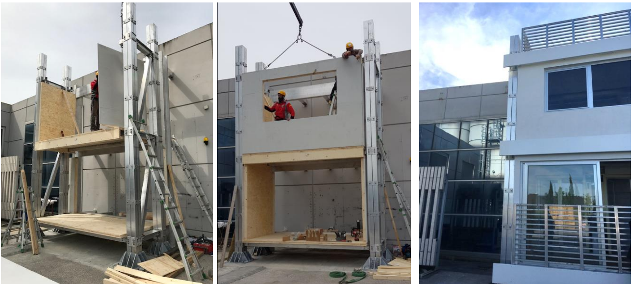
Figure 295 – Photos during and on completion of the mock-up of Pro-GET-onE in the ALIVA Srl plant – Source: [211]
