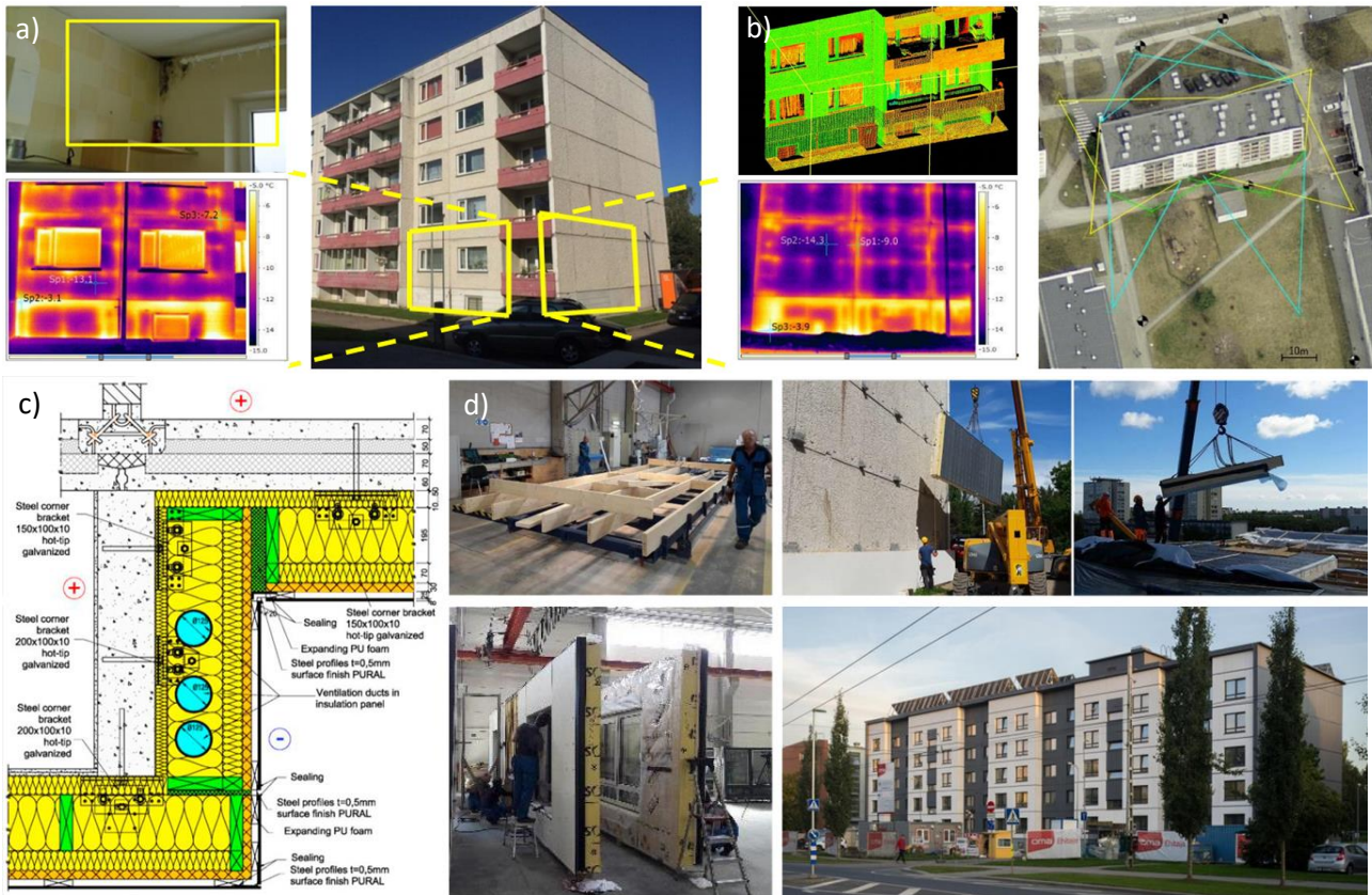
Figure 37 – a) Overview and thermal camera images of the MORE-CONNECT pilot building in Estonia before-renovation; b) graphic rendering of the laser scanner survey with indication of the shooting positions; c) example of designed solution with integrated ventilation ducts; d) photos of the production off-site of the panels, the assembly on-site and the final result – Source: [87, 89]
