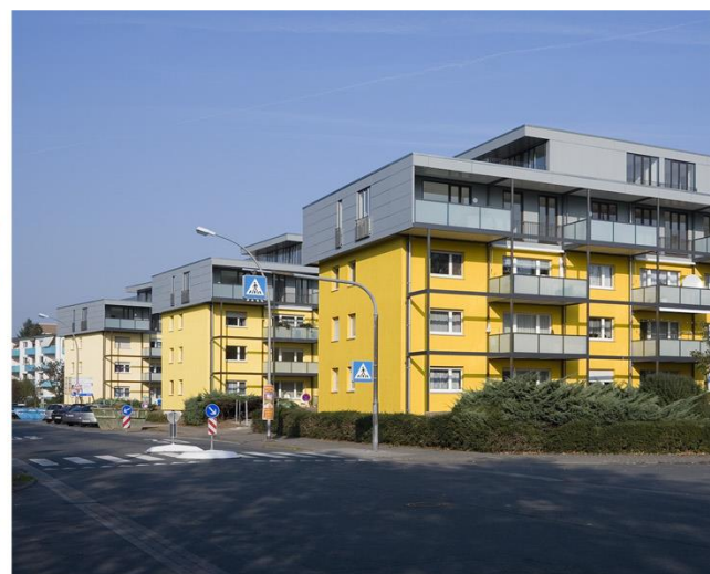
Figure 40 – Example of vertical extension with a floor-area densification ratio of 1.5, OPEL company owned apartments, Rüsselsheim – Source: [93]
