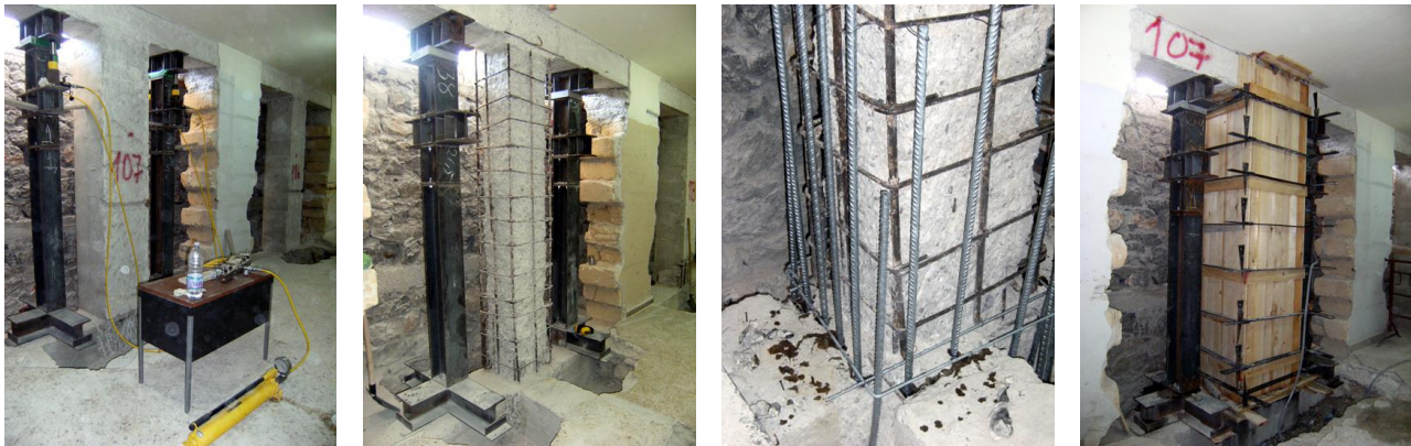
Figure 7 – Restoration of a degraded concrete column – Source: [28]
