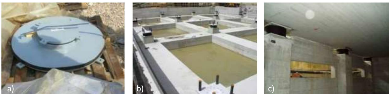
Figure 23 – Examples of isolator applications. A) One of the 12 isolators applied in the new school Francesco Jovine in San Giuliano di Puglia; b) some of the 61 high damping rubber bearing (HDRB) isolators installed at the base on the above-mentioned school; c) some of the 16 HDRB installed on an isolated floor of a building in Foligno (Perugia) – Source: [60]
