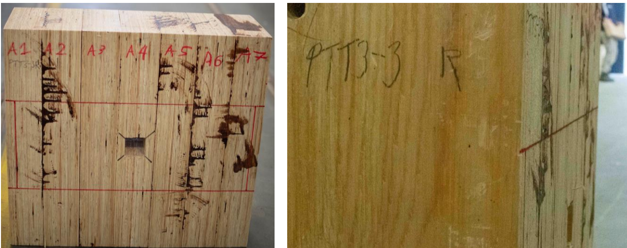
Figure 263 – Photos of the PTT3-3 wall sample after the test, no significant damage was observed (as for all similar samples)
