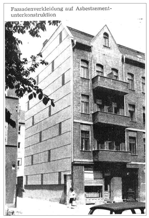
Figure 17: Asbestos cement panels for exterior cladding (Meier-Rouden [1975]: 27).
