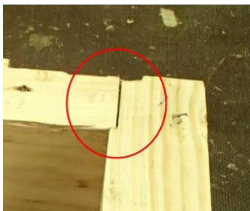
Figure 17: Deviations due to assembly inaccuracies.
