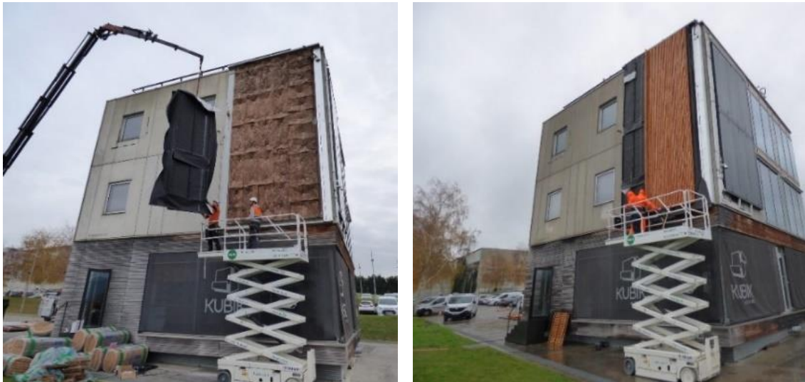
Figure 22: Installation of 2D modules using current techniques.
