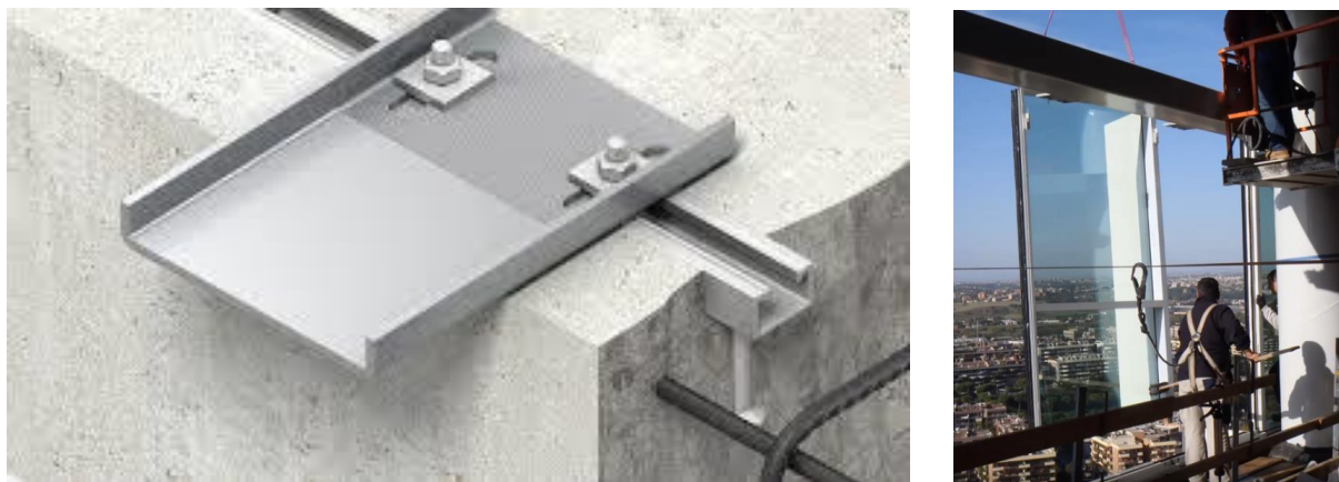
Figure 20: Installation of CWM Images courtesy of Focchi SpA.
