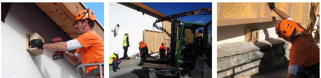
Figure 100: Installation sequence of the modules. The module below installed with a crane.
