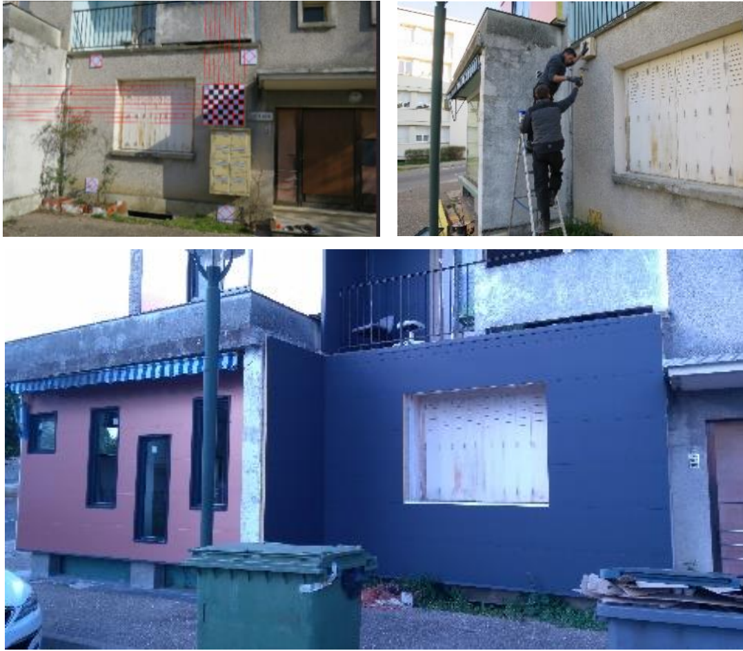
Figure 103: First achievements with photogrammetry and a module installed with an MK concept in a real project. Bottom picture by Mr Hervé Coperet (POBI Industrie).
