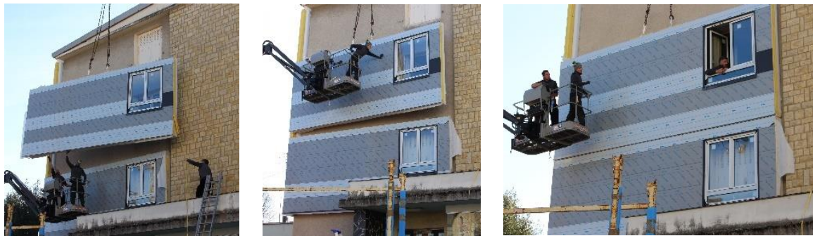
Figure 7: Issues while installing the modules in the BERTIM project [36].
