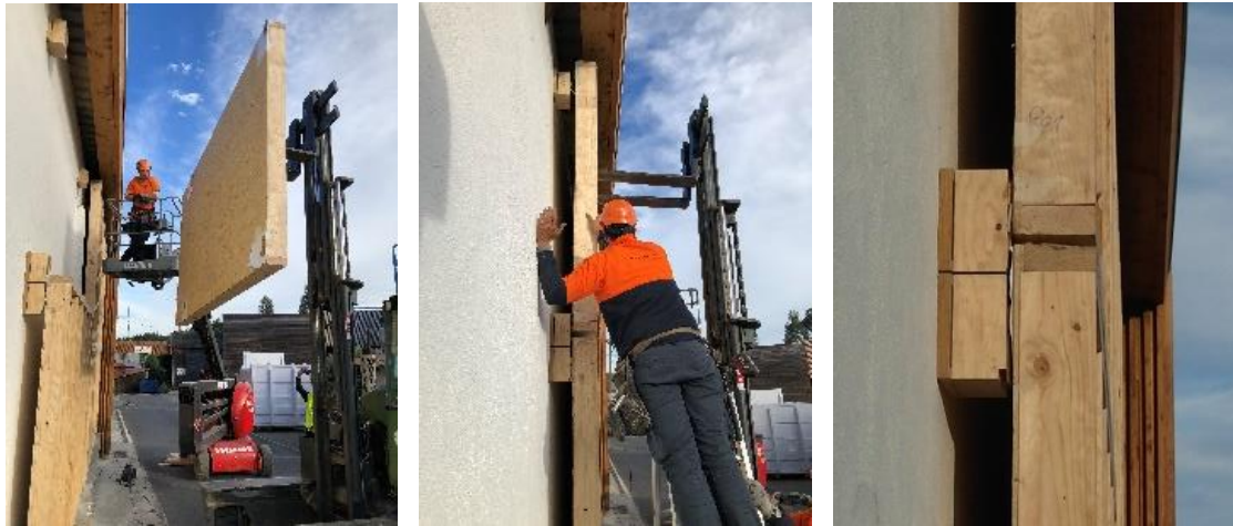
Figure 101: Installation sequence of the modules.
