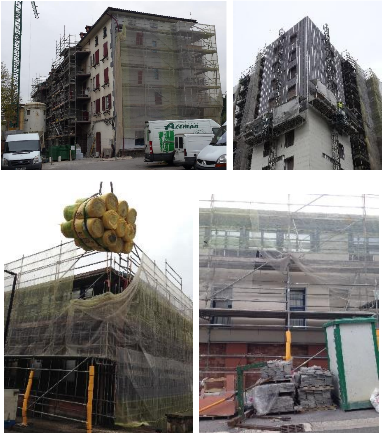
Figure 4: Manual techniques and logistics (Images courtesy of Artzamendi Eraikuntza S.L.).
