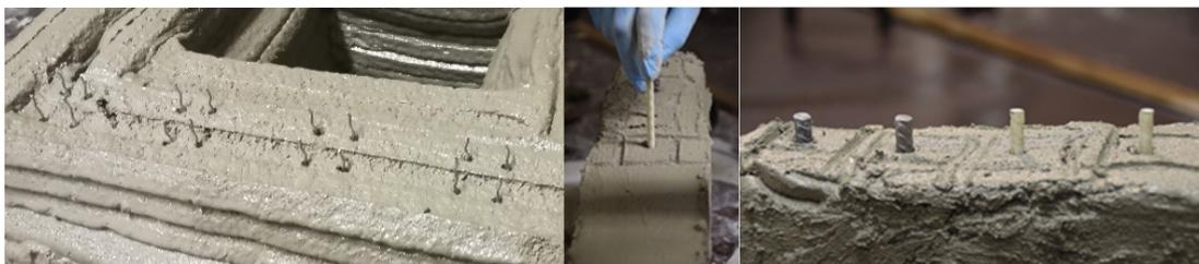
**Figure 3.** Vertical insertion of reinforcement: wire fibers (left), rebars (middle and right).
