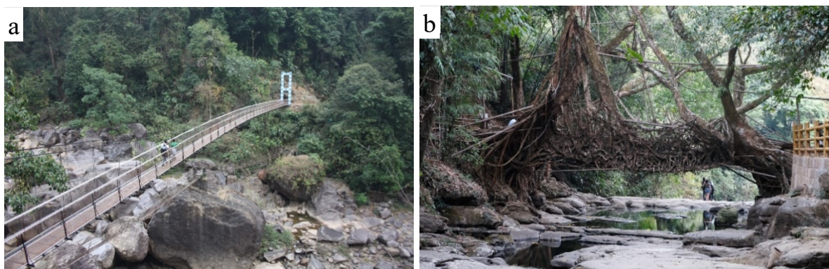
Figure 5. Two contrasting aesthetics: (a) The steel bridge towards Nongriat village can be described as modern, efficient, and professional; (b) the traditional Wah Thyllong bridge can be seen as an example of the Ecological Beauty of living root bridges (LRBs). The bank reinforcement and railing made of imported Cherra stone and painted reinforced concrete (imitating bamboo) illustrate a break with this tradition.
