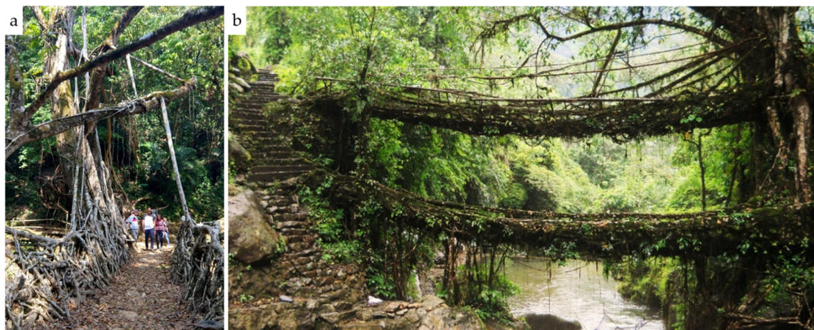
Figure 16. (a) Wah Thyllong bridge connecting Nohwet and Riwai villages has a wide and comfortable gangway. (b) A second deck was established on Nongriat Double Decker bridge. According to local residents, the upper deck was grown to allow the use of the bridge when the lower deck was flooded (photo: Patrick Rogers).
