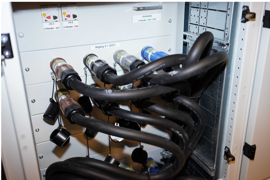
Figure C.3: View into the patch-panel system to configure the electricity grid
