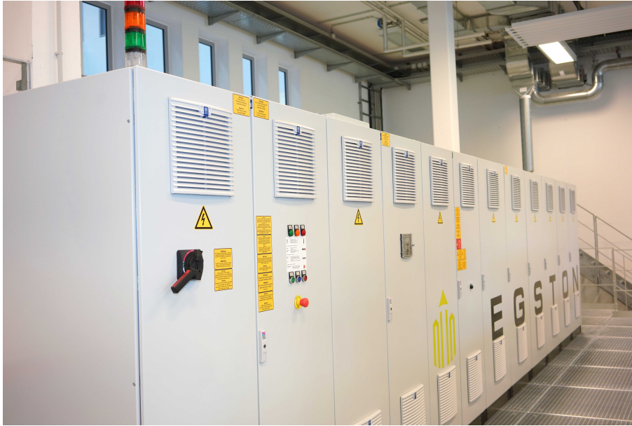
Figure C.4: Overview about the PHIL load emulator.
