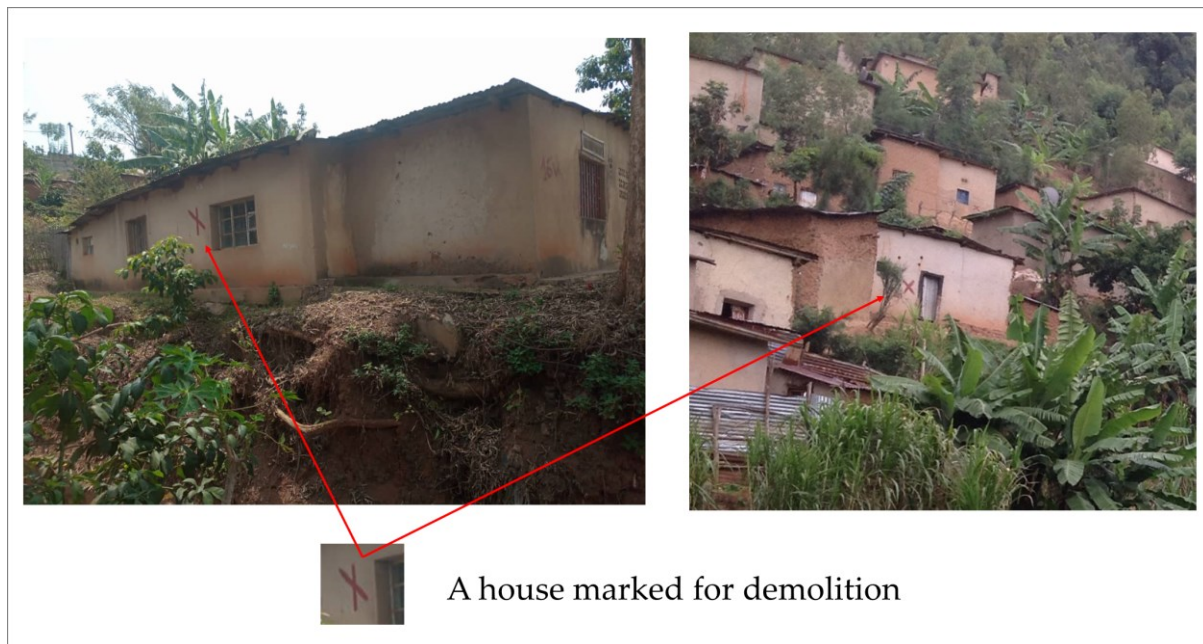
Figure 32: Houses in a high-risk area marked for demolition
