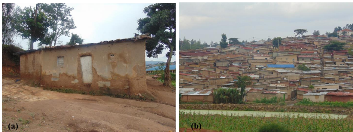
Figure 3. (a) Poor housing quality for the expropriated poor groups in Kangondo II; (b) Location of some of the expropriated residential buildings in the wetland area. Data Source: field observations.
