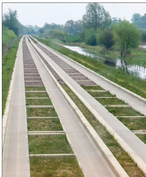
Figure 4-9: Cross section of Guided Busway Design in UK
