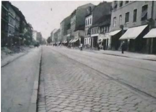
Figure 5 – Rosenheimer Straße (before)
