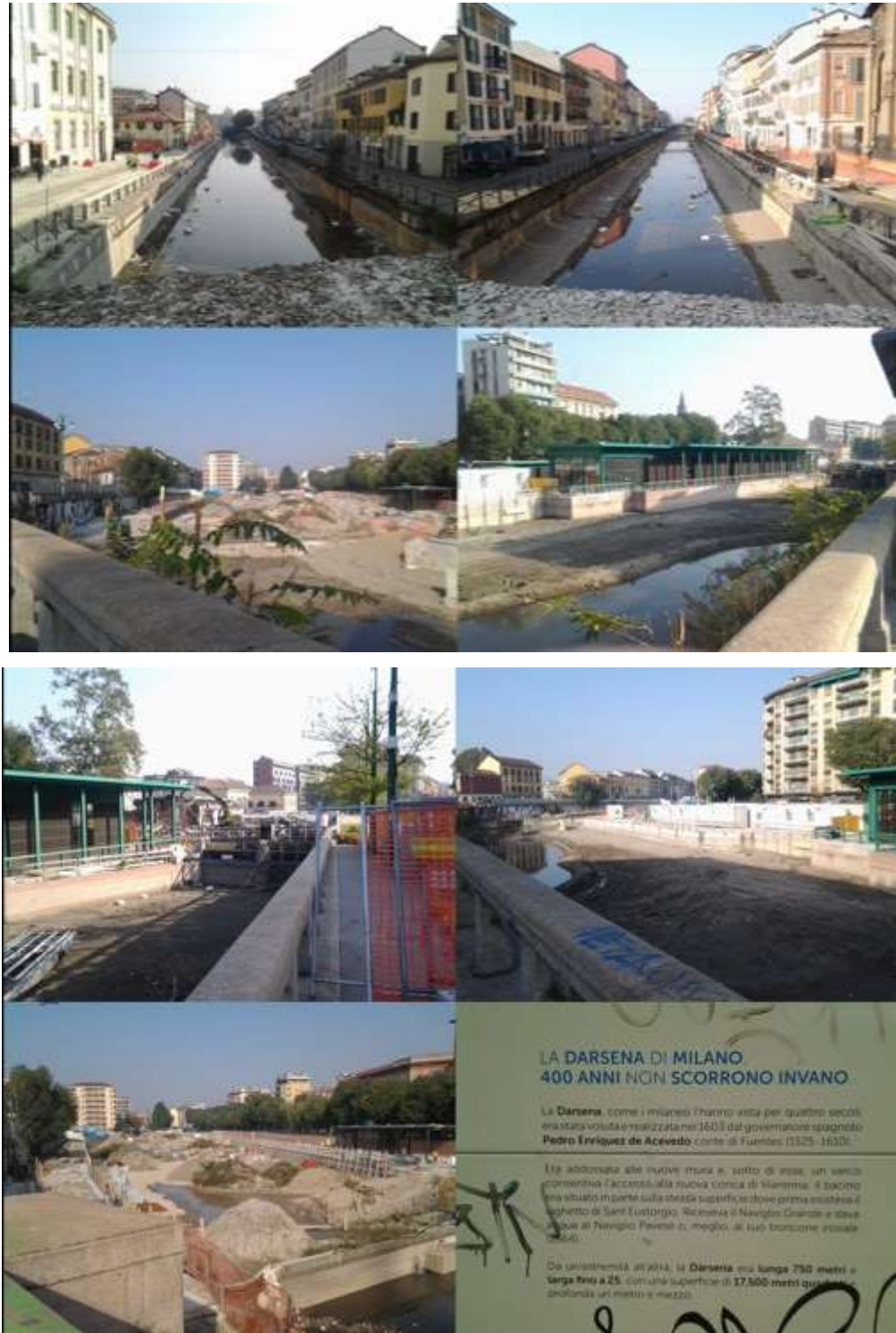
Figure 16. Darsena rehabilitation: state of work progress at 1.11.2014
