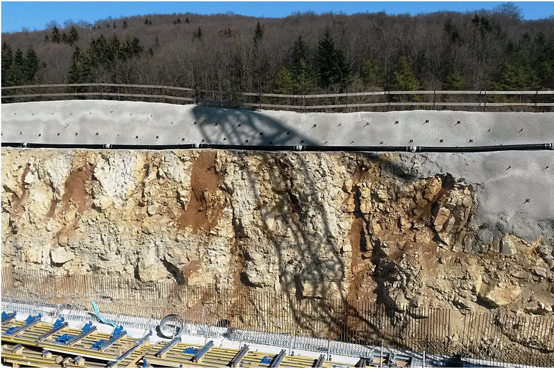
Fig. 5: Epikarst zone with partly highly weathered limestones. Imberg Tunnel, Swabian Alb high plain, southwestern Germany, 2016.
