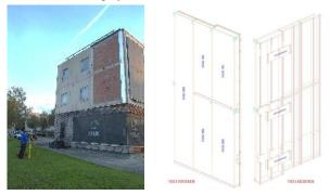
Figure 2. Left: Measuring the Kubik building strategic points. Right: Define the modules in CAD.
